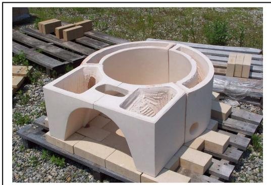
3) Set the entrance tunnel (2 pcs) and wall sections (2 pcs) as shown using HeatStop II refractory mortar.
